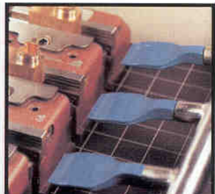
Blowing off portions of equipment machines
